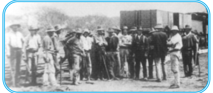
Workers awaiting the arrival of a trailer load of sleepers.
